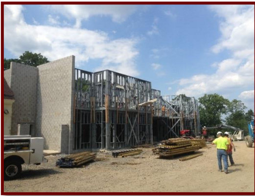
Figure 1.2 – East Wing Infinity Panels
