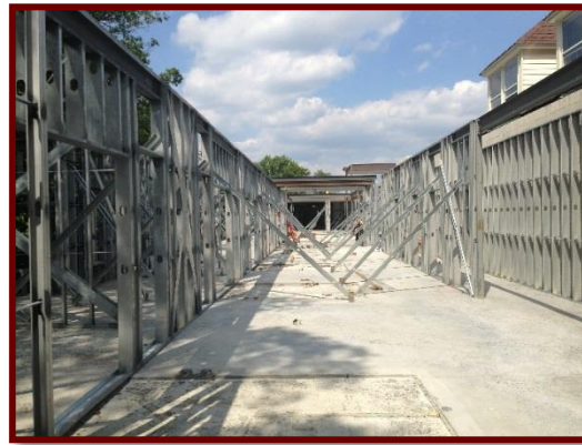
Figure 1.3 – Temporary Bracing for Infinity Panels
